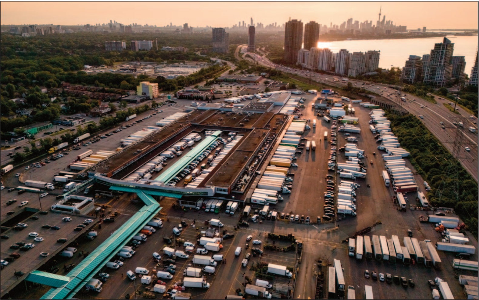
An early-morning drone shot of the Ontario Food Terminal shows the scale of the 40-acre distribution hub in Toronto. An expansion would see the farmers’ market come under a permanent, climate-controlled structure.
